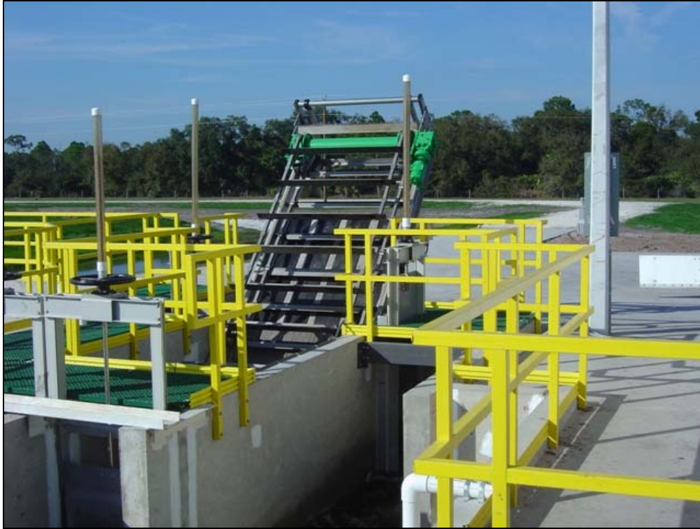
Illustration 5: Image of the TC-ATS Duperon FlexRake.
