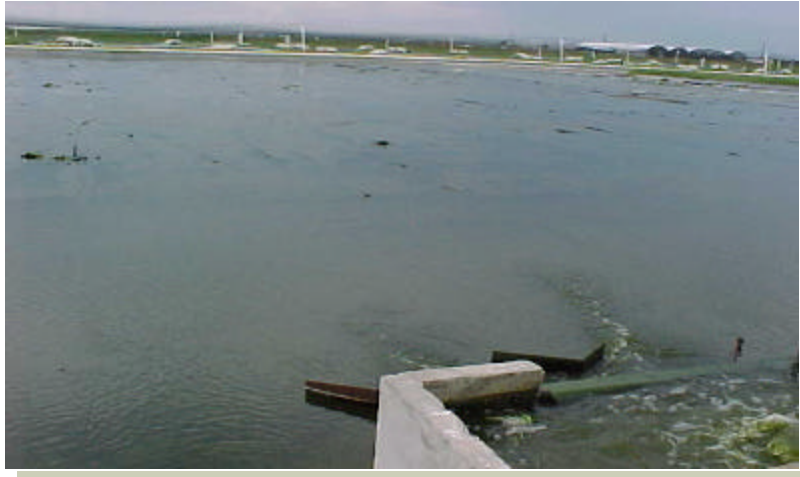
Algal Turf Scrubber (ATS) at Okeechobee, Florida fish production facility
