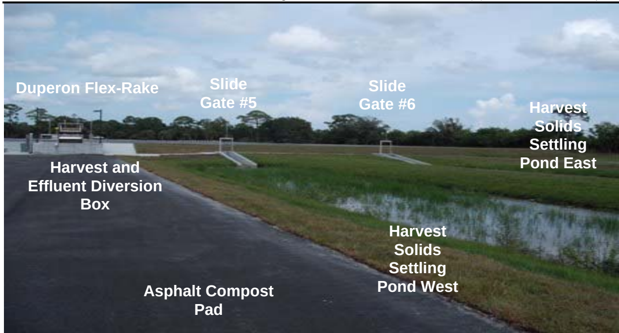
Illustration 13: Solids Settling Ponds which Receive Diverted Harvest Flows Containing Solids which Pass through the Flexrake
