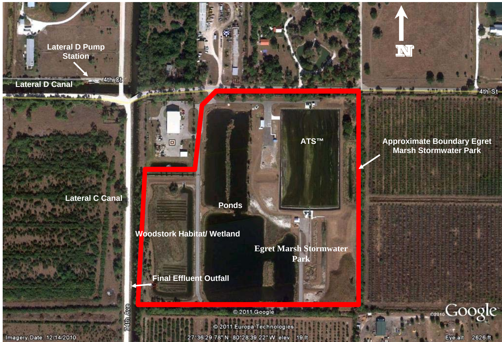
Illustration 6: Egret Marsh Stormwater Park Site Following Construction—Dec 2010
