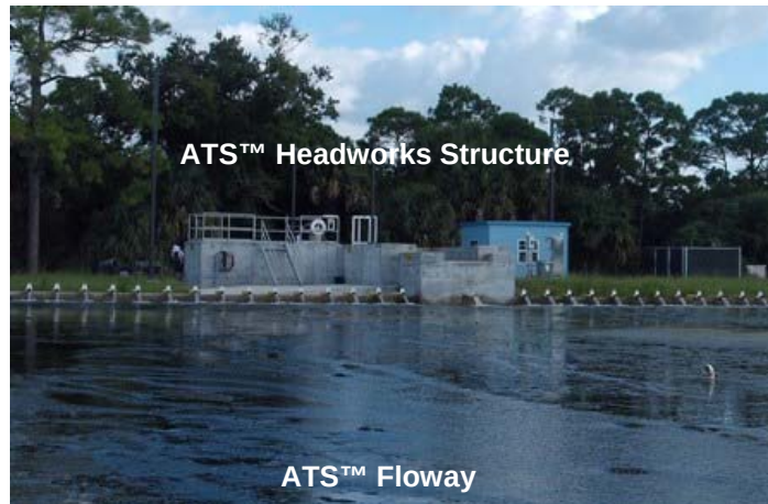
(a) Monitoring Station 01 (Looking North)
