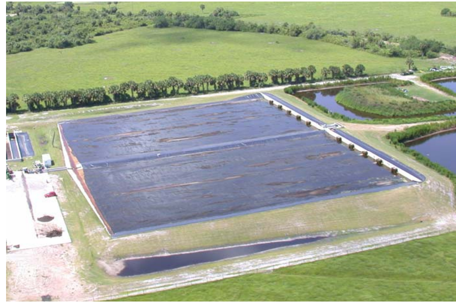
Aerial View of Algal Turf Scrubber®
