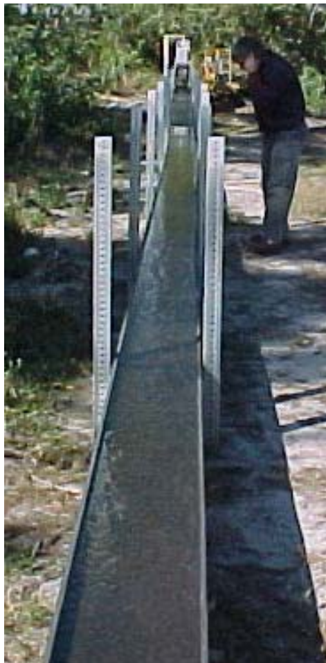
100' ATS™ MPU System Indian River County, Florida
